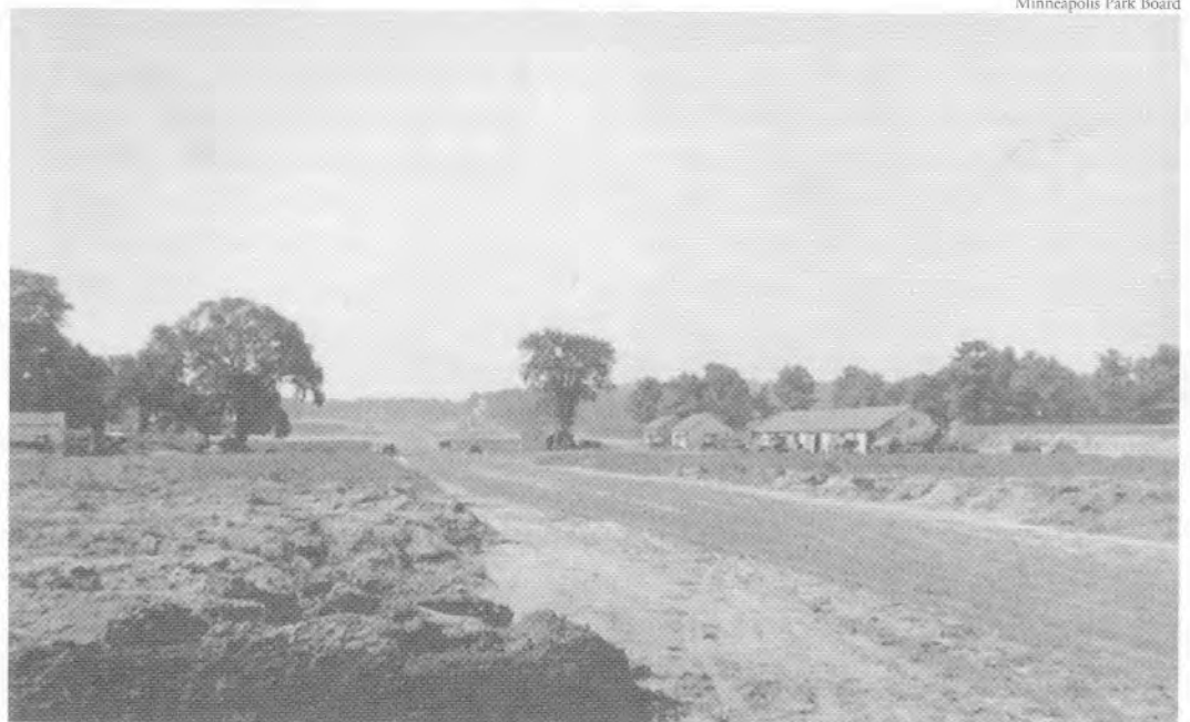
Construction of the parkway, completed in 1921, cost approximately $385,000.
