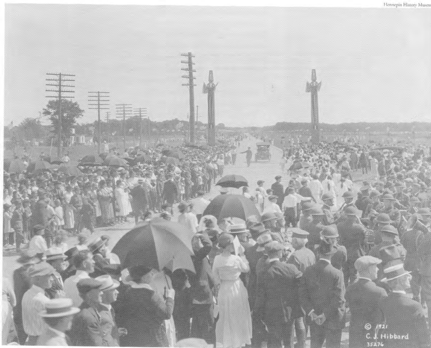
More than 30,000 people assembled in the northwest corner of Minneapolis on June 11, 1921, for the formal dedication of Victory Memorial Drive.
